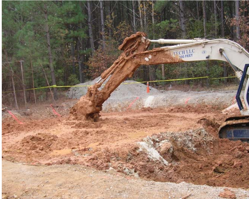
Figure 3: In-situ Blender Mounted on Excavator during Soil Mixing Activities
