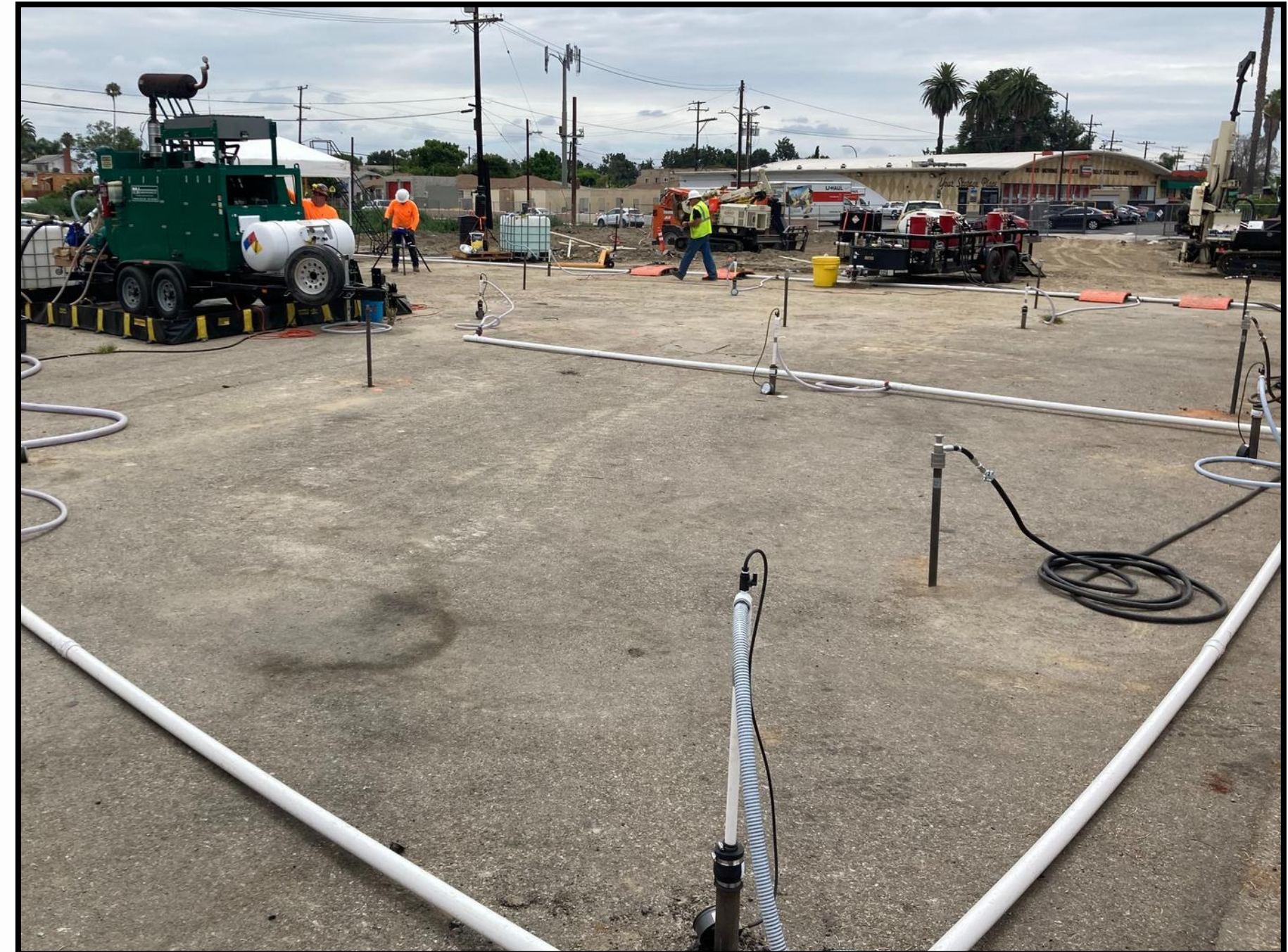
Placement of temporary extraction locations and steam injection locations
